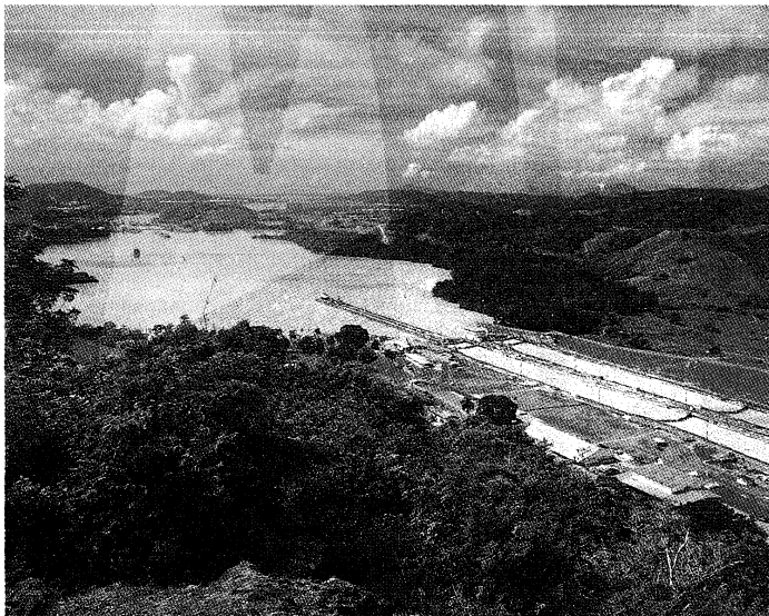
The Pedro Miguel Locks raises or lowers ships on the Pacific side of the Panama Canal.
