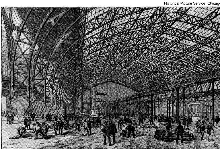
Figure 7: Steel and glass construction using three-hinge arches, the Gallery of Machines, Paris, 1889 (demolished 1910).
